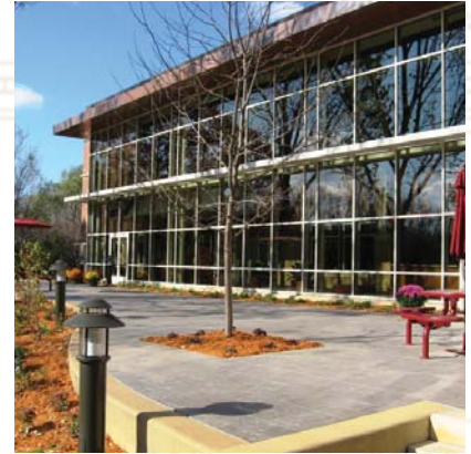
Woodbury City Hall, Woodbury, MN
