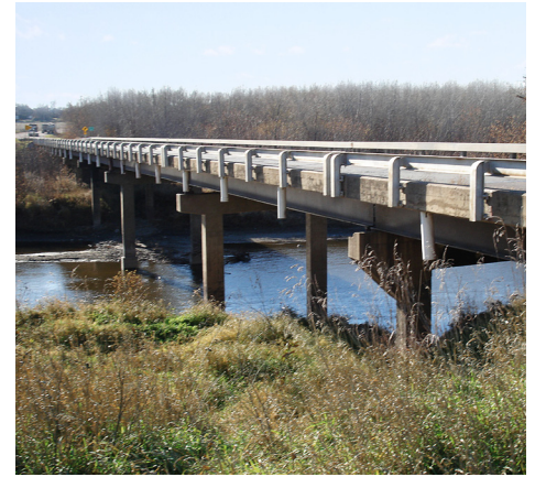
Steel Girder Bridge Hudson, SD
